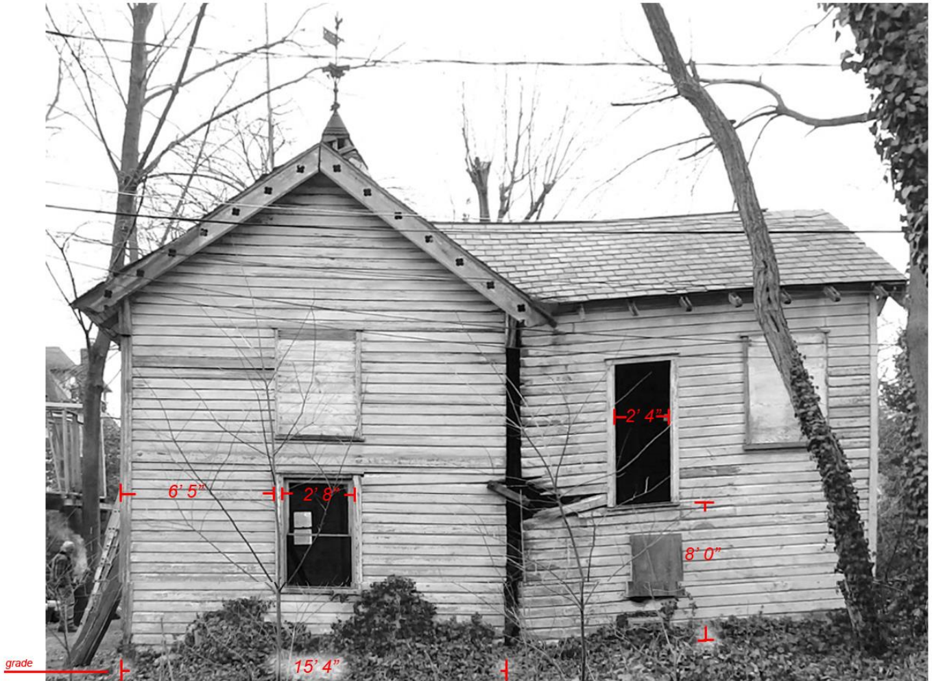
Looking toward Main St. Clothier Carriage House, 3rd and Main, Riverton, NJ February 2017
