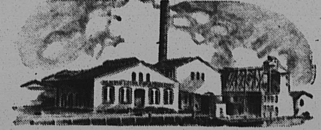
AN ELECTRIC GENERATING STATION ABOUT 1903
