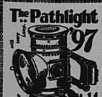
lights the way and stays lighted. All brass, nickel plated—no thu; outside oil-filler; cotton packed oil fount; double convex ground photolens; burns ferosene, throws a light 60 ft. and weighs but 12 ounces.
