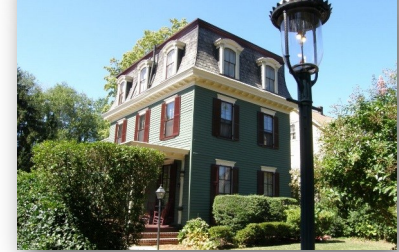
404 MAIN ST. (top) and 402 MAIN ST. (bottom)
